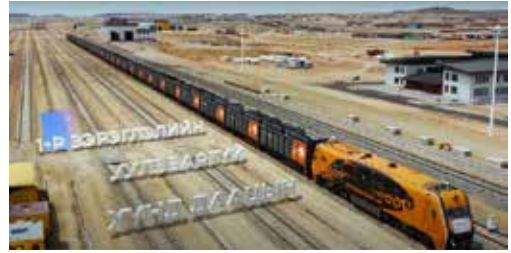
TAVANTOLGOI - GASHUUNSUKHAIT RAILWAY COMPLEX PROJECT
